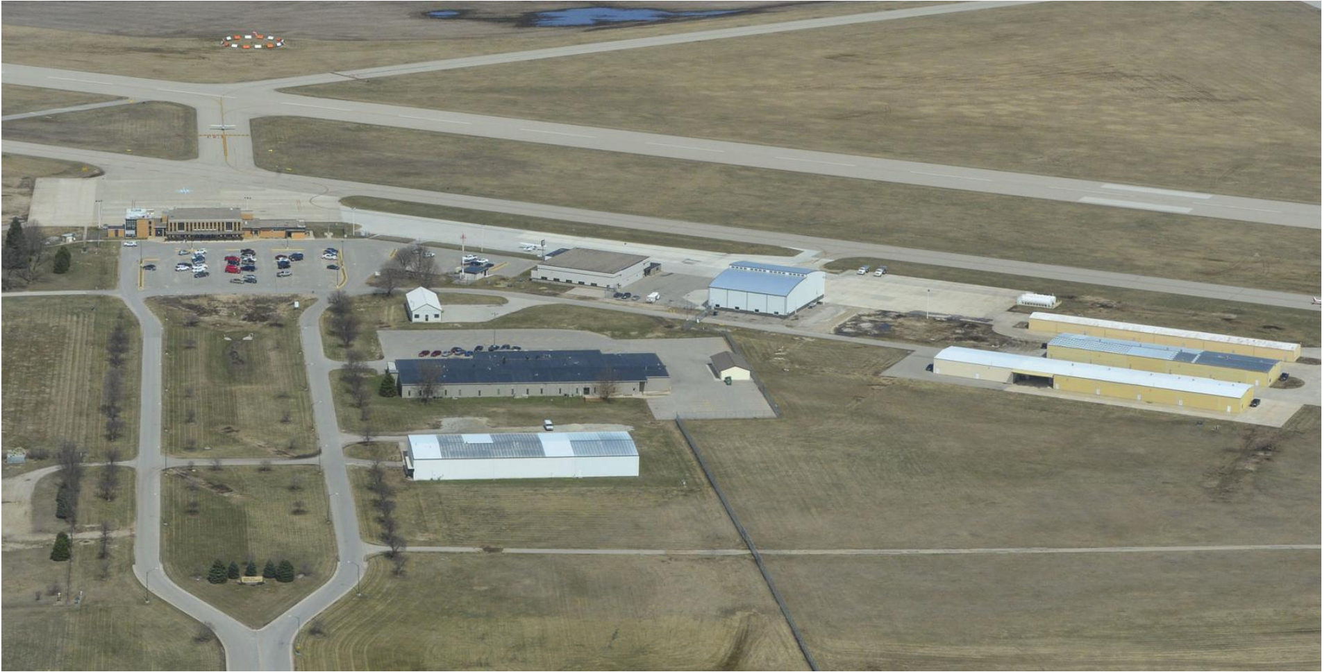
Mason City Airport
